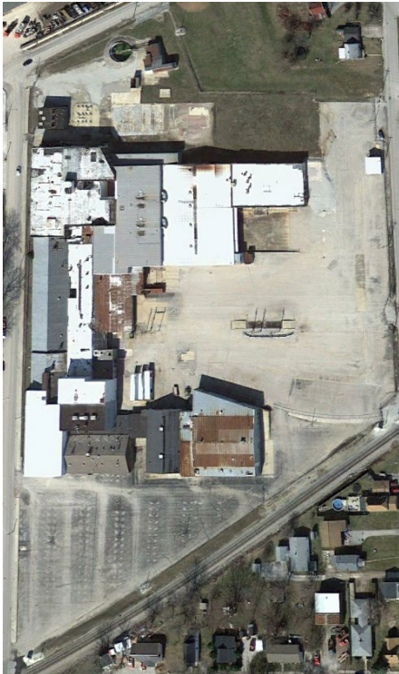
Image: 1 An aerial image of the former Exide Technologies Facility site, Pre-Demolition, Circa 2012.
