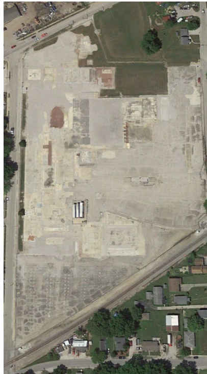
Image: 2 A recent aerial image of the former Exide Technologies Facility site, Post-Demolition.
